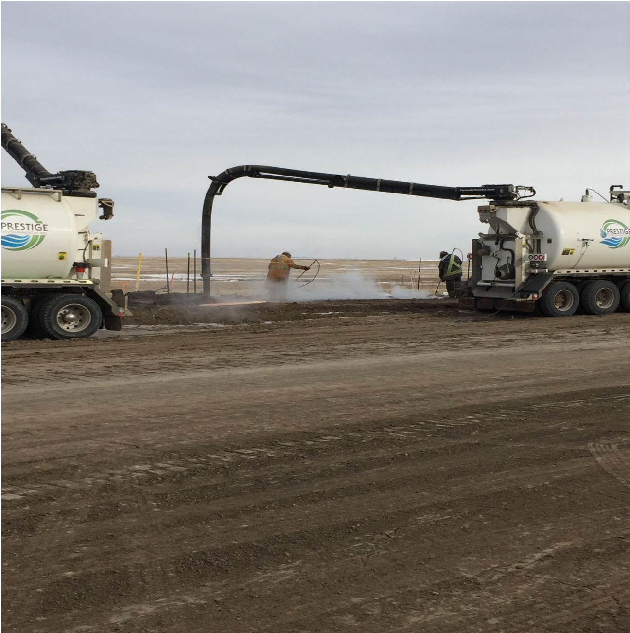
Hydrovacs exposing existing lines before trench is dug.
