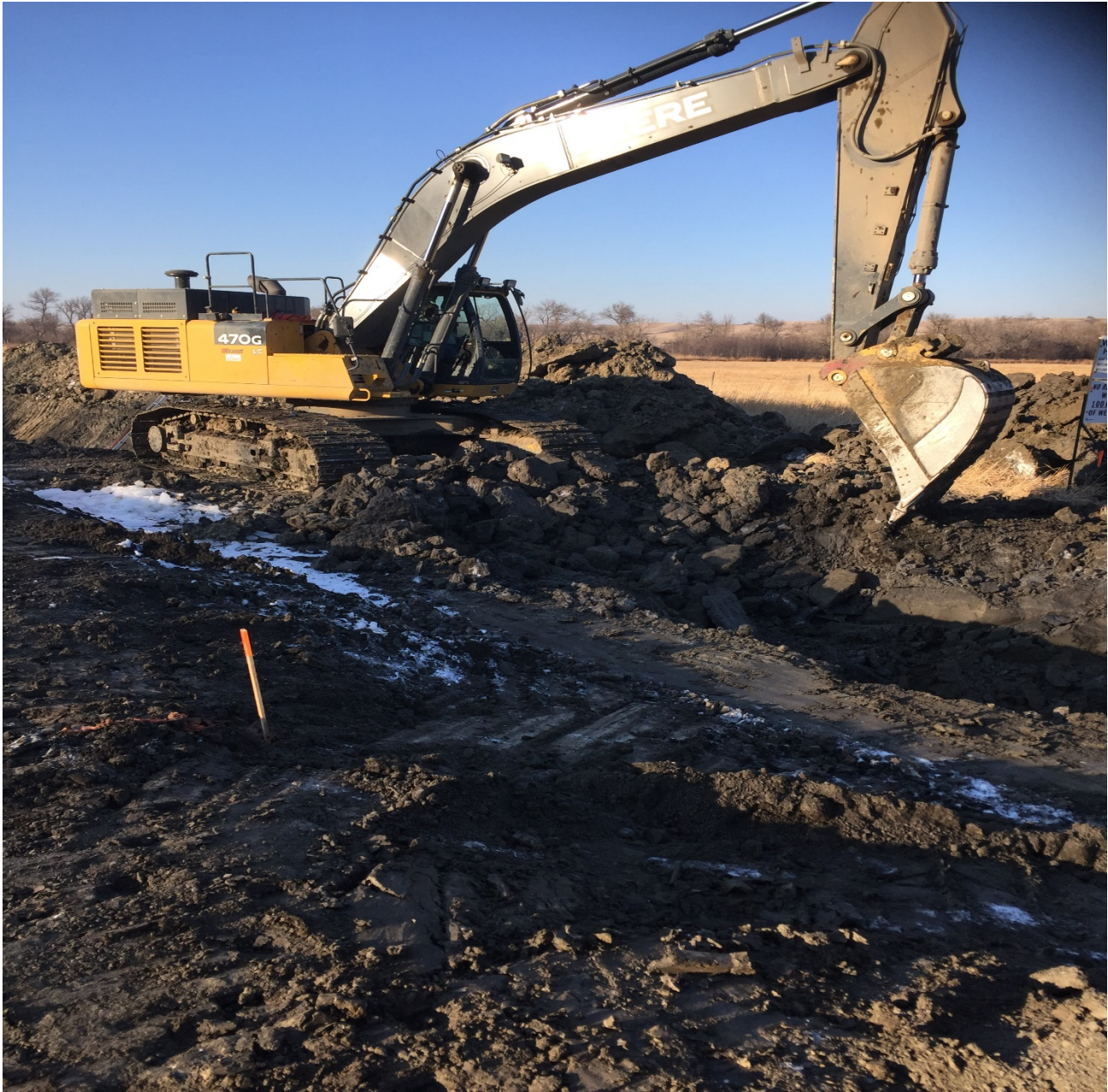
Excavator backfilling trench with pipe in the ground.
