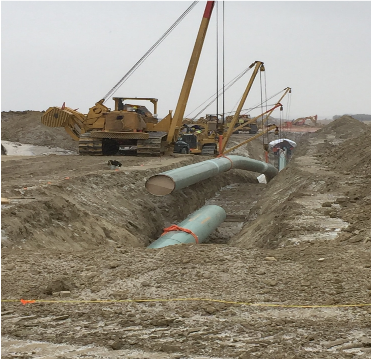
Side booms connecting tie-ins and welding to existing pipe in trench.
